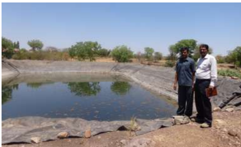
Fig.1 Farm pond constructed under the scheme Farm Pond on Demand implemented Govt. of Maharashtra
