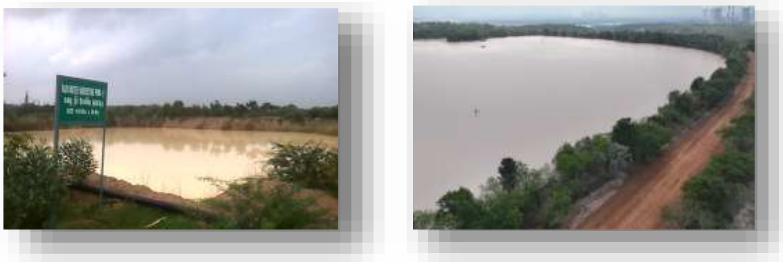
Fig.8 Rain water harvesting pond in NLCIL
